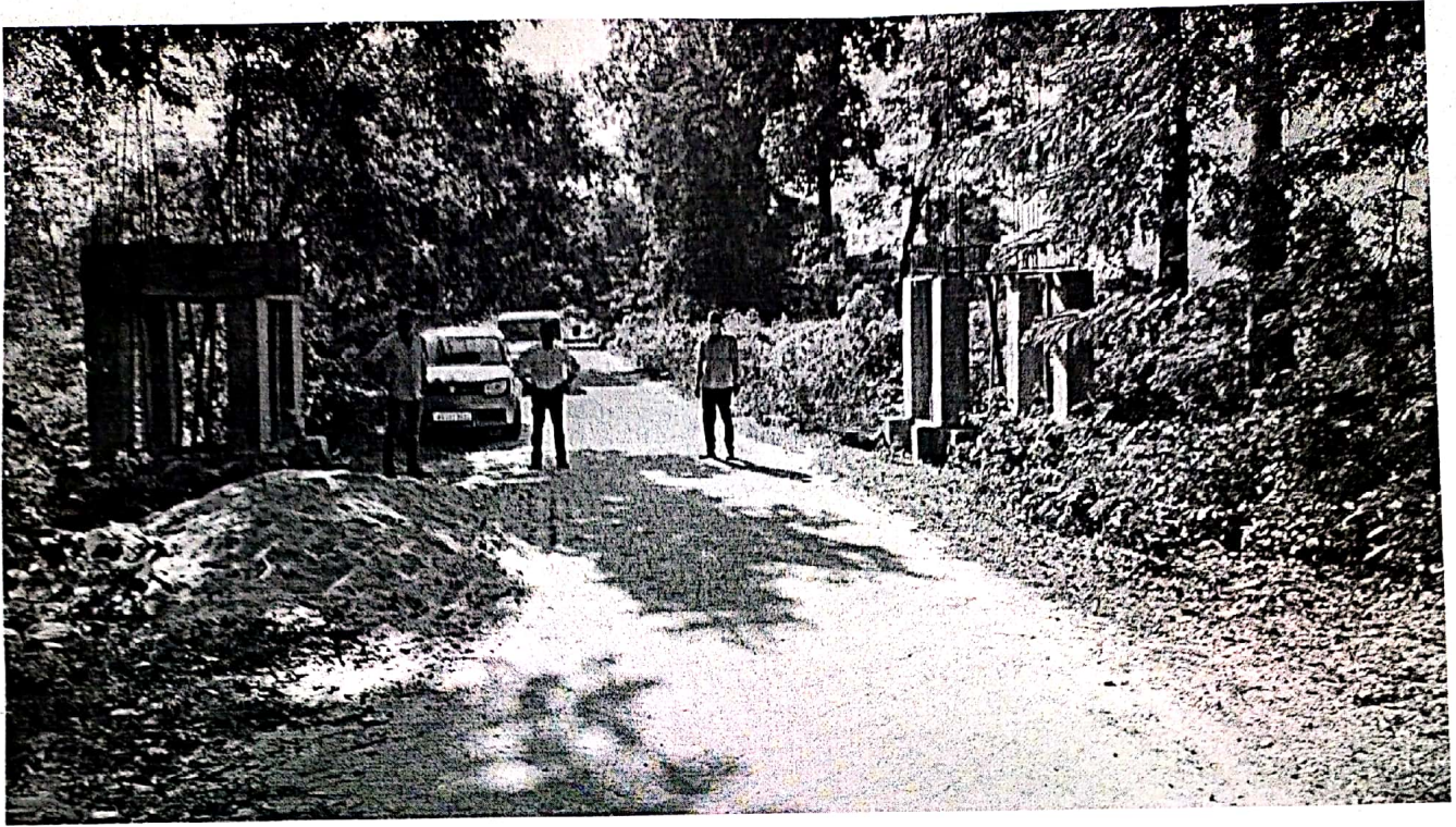
Construction of Welcome Gate at Village Kadamani
